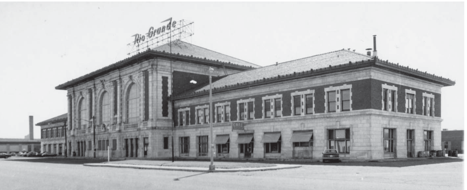
Denver & Rio Grande Depot. Photo Courtesy of Utah State Historical Society.
