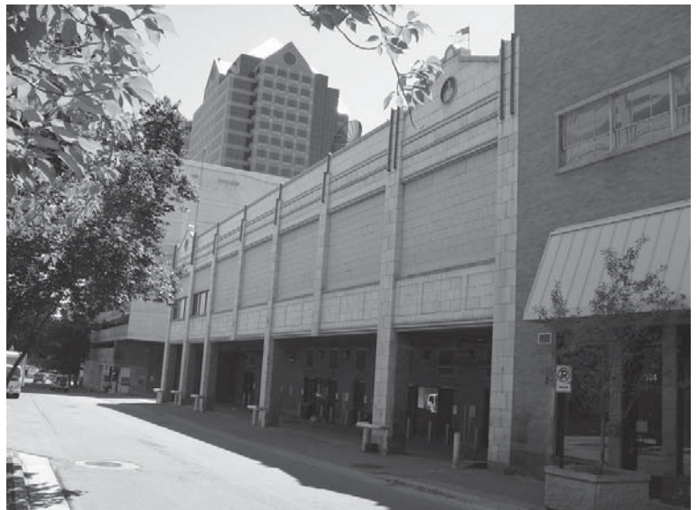
Salt Lake Tribune Printing Press Building located on Regent Street (50 E). Slated for Demolition in January 2014.
