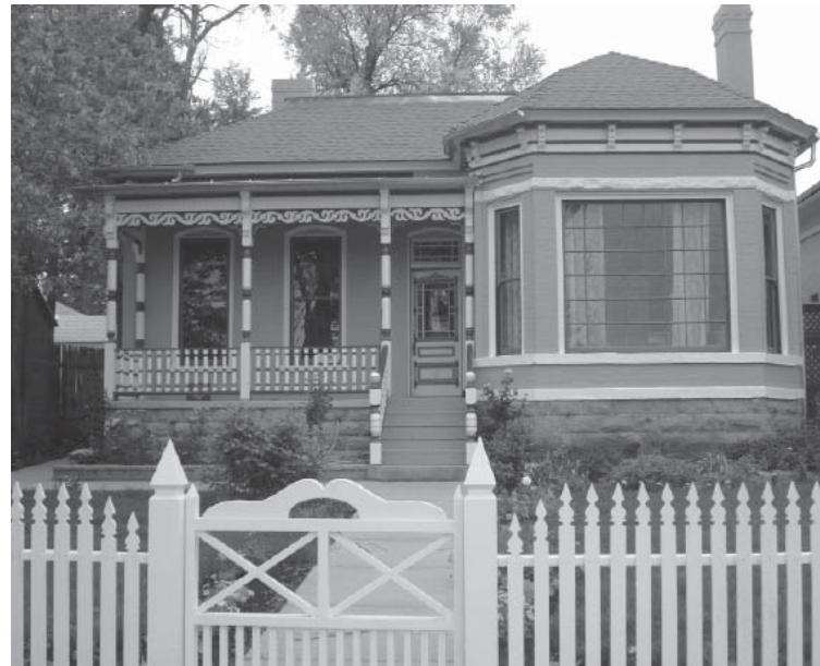
The Romney House after the Carlson's renovation.
