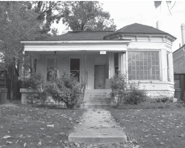
The Romney House prior to renovation.
