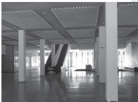
The first floor interior remains pristinely open with original floorplan, light fixtures, and colors intact.
