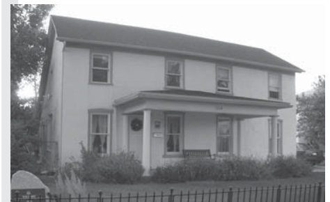
Wilford Woodruff's farmhouse is partially a log cabin that has been covered with stucco.
