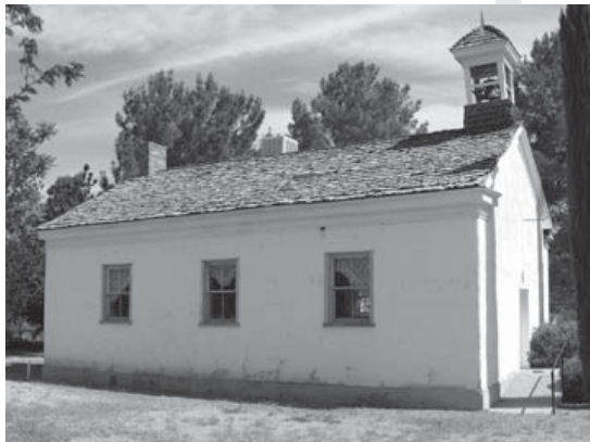
The residents of Virgin, Utah will use this 1866 adobe LDS meeting house as a community center after its restoration.
